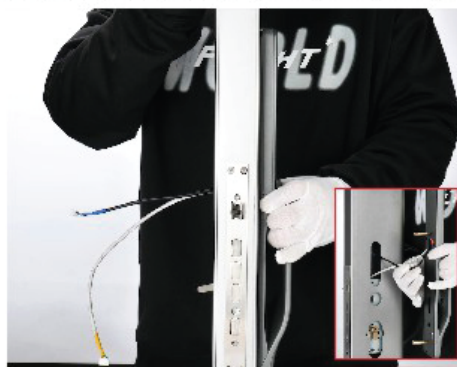
14. Before installing the lock, note: first pass the data cable through the door hole
