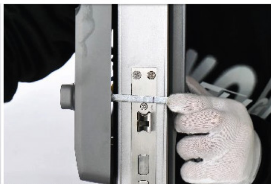
20. Trim the length of the deadbolt tail according to the door thickness, ensuring it does not exceed the outer door edge.
