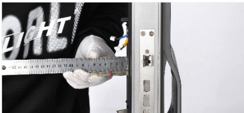
19. Measure from the edge of the door to the square rod, leaving a length of 25mm to 35mm, make a mark, and cut of the excess part. 20mm, make a mark and cut of the excess part.
