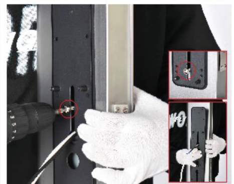
15. After installing the lock gasket, screw in the bamboo-shaped screw but do not tighten it to facilitate later adjustment
