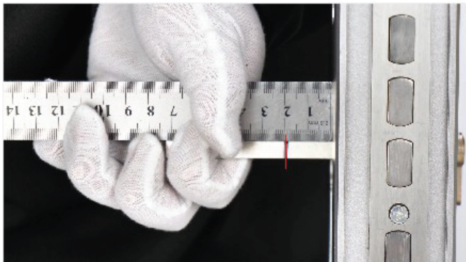
11. Measure the tail size on the lock cylinder. According to the door thickness, the tail size on the lock cylinder should be 18mm to 20mm. Mark it and cut off the excess part.
